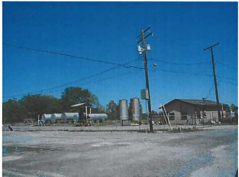
Above ground storage tanks near Site 4
